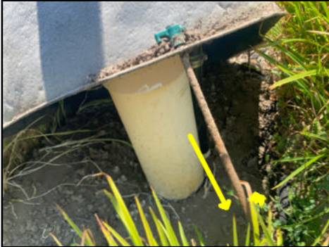
Location of the wellhead
