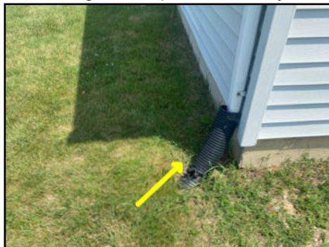
Maintain underground drains
