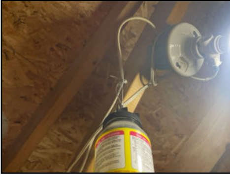
Extension cords should not be used for permanent wiring
