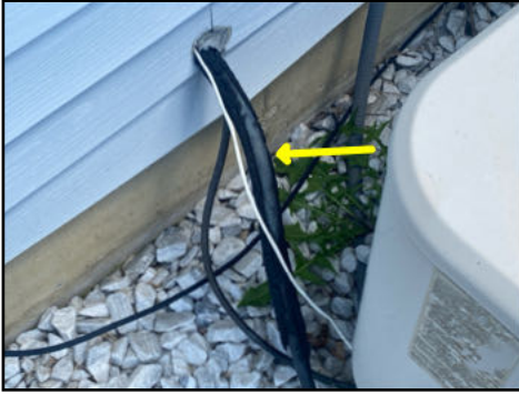
Deteriorated/missing insulation
