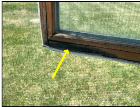
Moisture stains/damage
