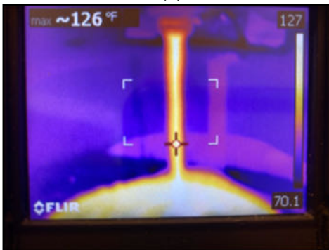
Hot water temperature at the hallway bathroom sink
