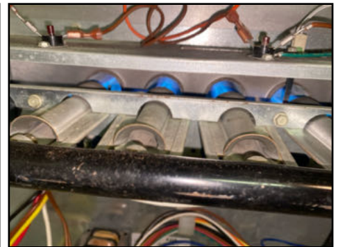
Burner operation
