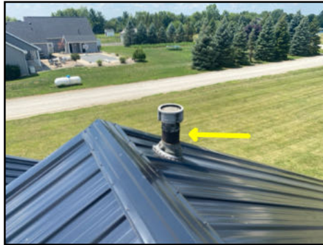
View of the furnace flue
