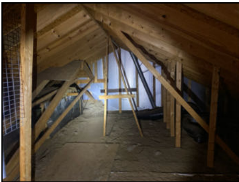
View of the structure
